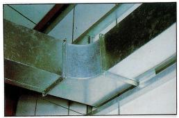
Acoustic Turning Vanes can be substituted for existing ducted bends with no space penalty.
